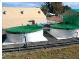
Prefabricated FRP Tank
