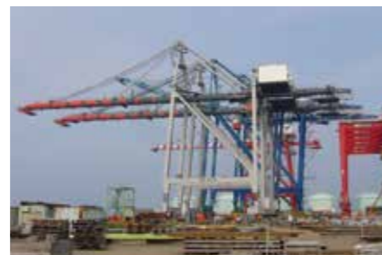
Harbor Container Crane
